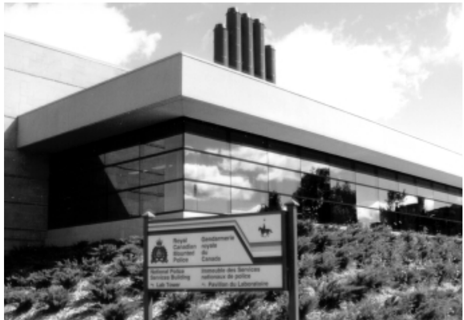
Canada's national DNA Data Bank at RCMP Headquarters in Ottawa.
